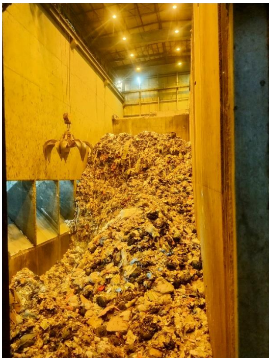
Bromley's non-recyclable waste co-mingled with Lewisham and Southwark (the bottom picture !)
